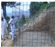
Work in progress on Drinking Water Supply Scheme in Dir Upper
